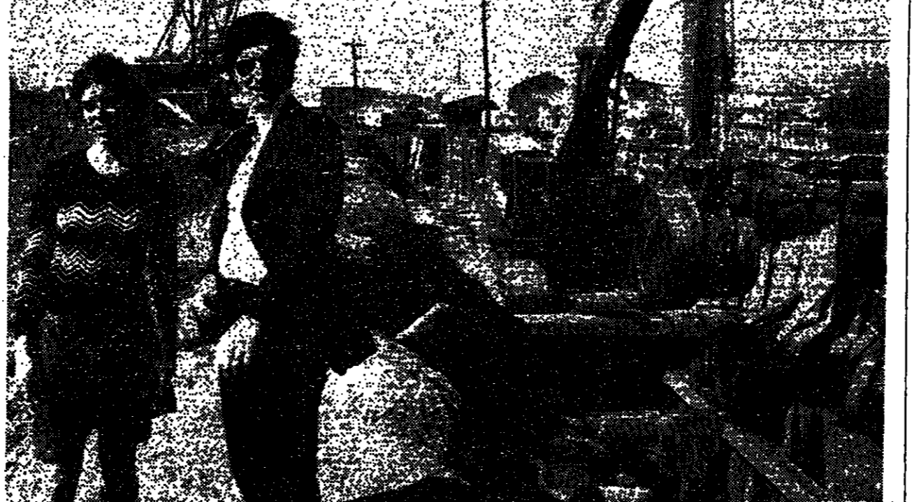
Robert J. Mrzak, chairman of Suffolk Legislature's Finance Committee, and Lisa Riordan, legislative aide, at sewer construction site in West Islip, L.I. They contend much of the system already installed is defective.
